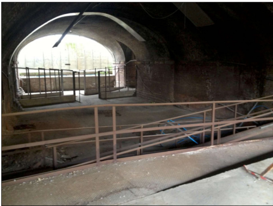
EXAMPLES OF VARIATION IN FLOOR LEVEL AND FINISH - Existing condition to be excavated/filled to facilitate level access to all areas from London Road.
